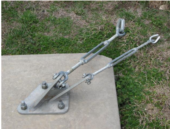
7/8" turnbuckle furthest from tower 5/8" turnbuckle closest to tower
