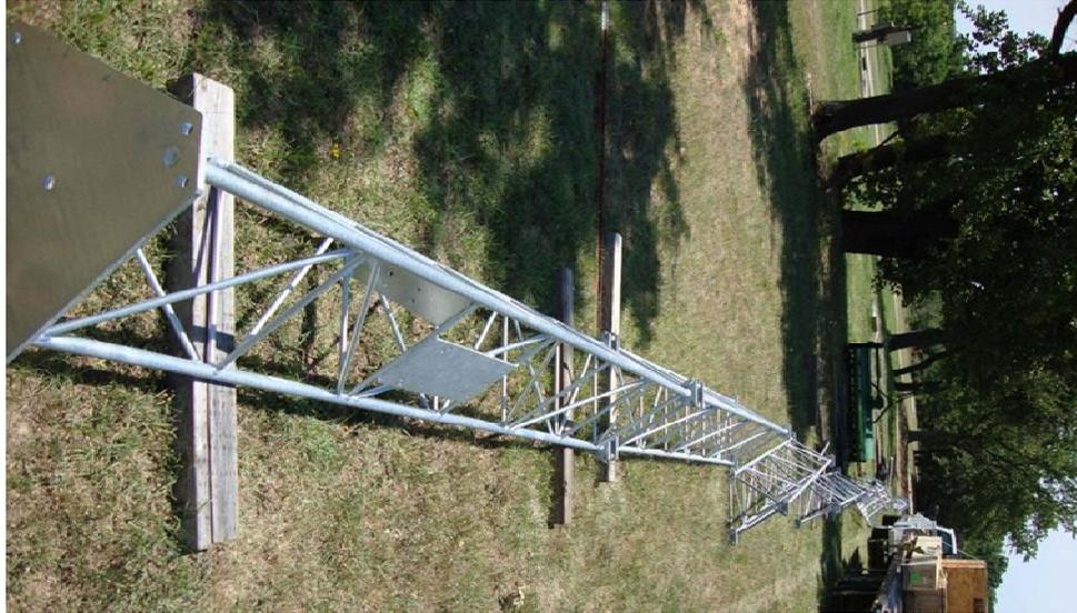
For 60'-140' towers, lay out the tower sections in a line so that the lift point of the tower is roughly lined up even with the base pad. The sections should provide a continuous lattice pattern. *Orient the base section to allow easy access to the disconnect attachment plate.*
