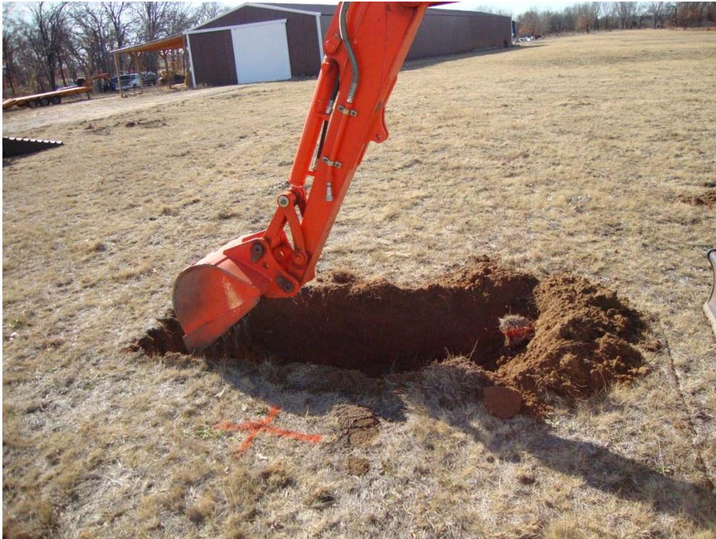
Dig a hole of appropriate size and depth, oriented perpendicular to the GR line. The **front edge** (towards the tower base) of the hole is the reference point for measuring the required anchor radius (**guy radius + 6 ft**). This job is best done with a backhoe.
