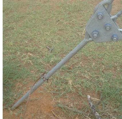
29. Ground the tower, switch box, and guy anchors with the copper-clad ground rods and special hardware provided in the tower hardware kit. If the rods cannot be driven in the full 2.5m (8 ft), it is advisable to drive extra rods and connect them. Another strategy for grounding in rocky soil is to lay the rods horizontal in a trench. No matter what grounding bar orientation is used, it is important to have the rods in moist soil for effective grounding.
