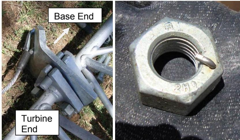
Joints that include guy tabs use 3/4” bolts that are 3.25” in length and heavy “Pin-Loc” locking nuts. A PAL nut is not required where a Pin-Loc nut is used.
