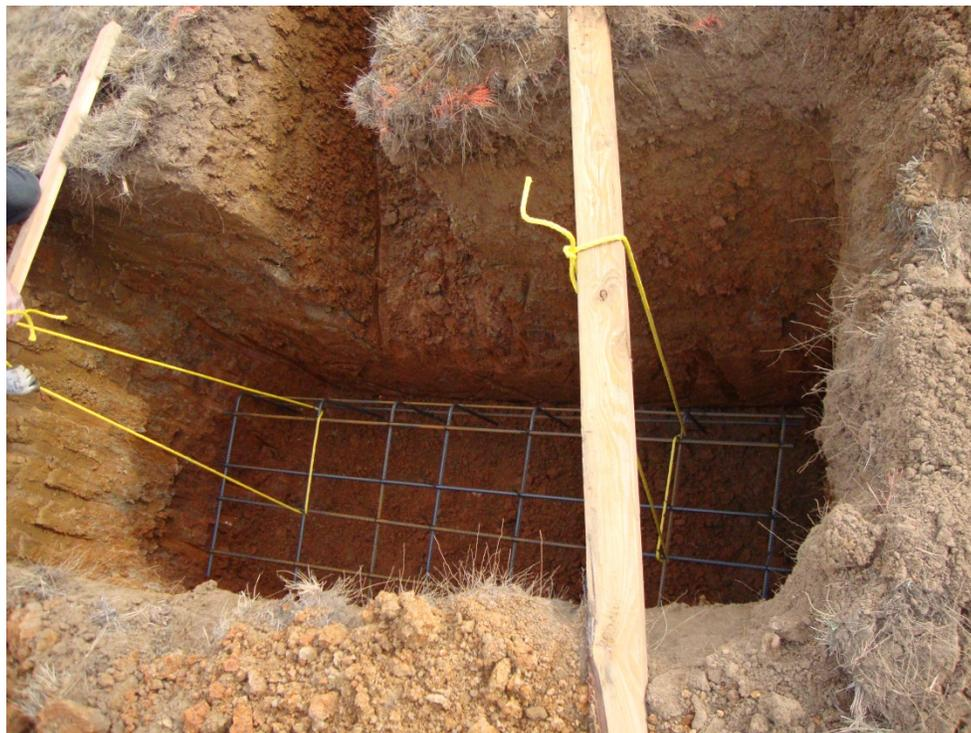
Prepare three reinforcing bar “cages”. Suspend the cages so that an appropriate amount of clearance is provided. Pass the anchor rod eye through the rebar cage, and then place the cage and rod in the hole so that the rod sits in the slot and the plate is centered in the cage. Check the angle of the anchor rod and support it so that it rests at ~45° above horizontal (55° for 140-160 towers).
