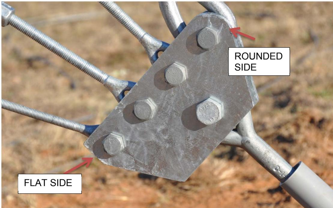
A different equalizer plate is used for 160' towers. This plate has a 4-hole configuration. When assembling the plate, remember that the flat side of the plate goes down, while the rounded side goes up, as illustrated in the previous picture.
