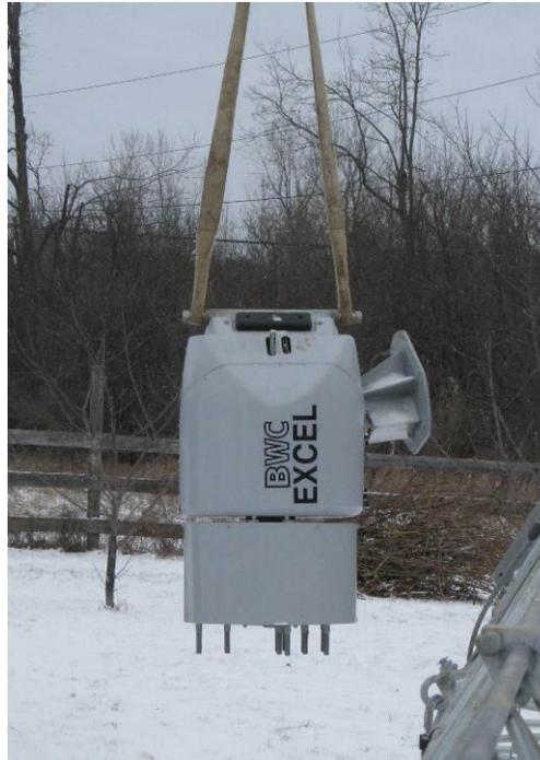
6. Use the crane to lift the powerhead, still attached to the shipping skid, clear of the ground using a double-eye nylon strap. Slip one eye over each end of the tail pivot pin and onto the mainframe; hook the crane line to the center of the strap and lift. The shipping nuts can now be removed from the blade studs so the skid can be pulled off and set aside (Excel 10k shown).
