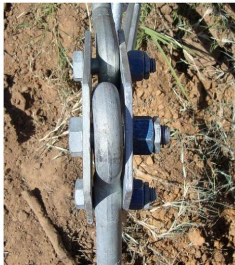
Tighten the 5/8" bolts for the turnbuckles to the point that the equalizer plates are parallel.
