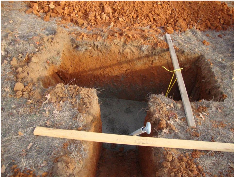
**NOTE:** Make sure the oval-eye at the end of the rod is positioned vertically so the equalizer plates will be vertically aligned when installed.
