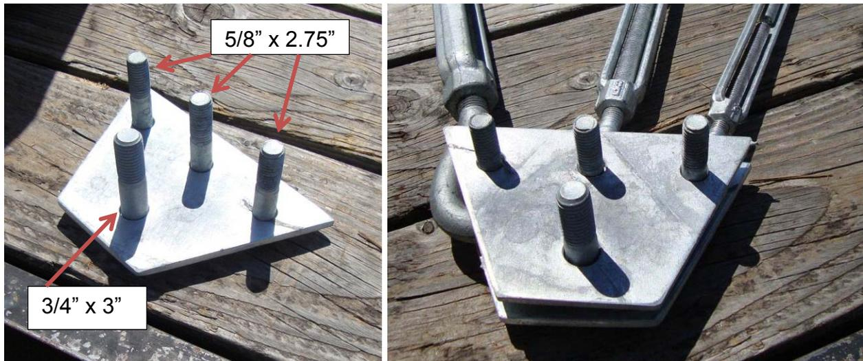
Assemble the 3-hole equalizer plates and turnbuckles, with one of the “eyes” of each turnbuckle attached between the equalizer plates. The 3/4” turnbuckles always go in the top 5/8” bolt hole. On 60’ – 100’ towers, only two guy levels are used so the middle 5/8” bolt hole on the equalizer plate is left empty. The 3/4” bolt hole is used for the anchor-equalizer plate connection.
