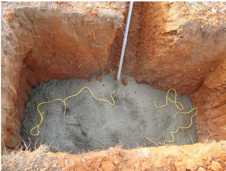
The concrete shall be placed in direct contact with undisturbed soil; using a vibrator to be sure it fills properly around the rebar and anchors.
