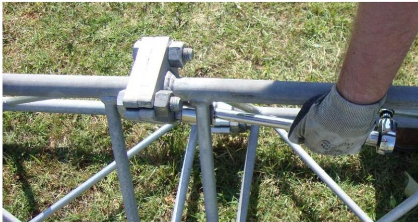
Once the tower has been put together, **use a torque wrench** on all connecting bolts. *The proper tightening torque on all section coupling fasteners is **205 ft-lbs**.*
