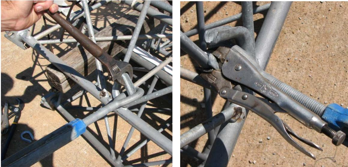
Once the eye has been slipped into the opened thimble, close the thimble. If you are having difficulties opening the thimble, it may be a good idea to secure the thimble to the tower crossbar with a locking wrench.
