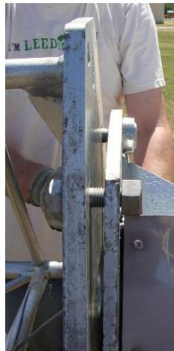
7. Direct the crane to move the powerhead until the tower adapter plate meets the tower top plate. Use one or two spud wrenches to line up the six attachment holes on the two plates. Bolt the turbine in place using 6 bolts, 3/4"x3-1/4", with hex nuts, PAL nuts and washers as required. Remember - **nuts go on top!** This hardware is included in the tower hardware kit (Excel 10k shown). Use the turbine mounting spacer provided as necessary, to be sure there is enough bolt thread to allow full
