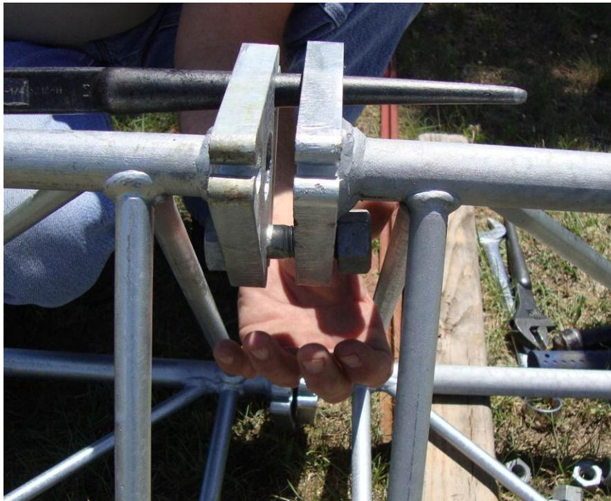
A spud wrench, 18" or longer, can be useful in aligning the flanges of the sections being bolted together. It is recommended to connect the bolts on the inside of the tower first.
