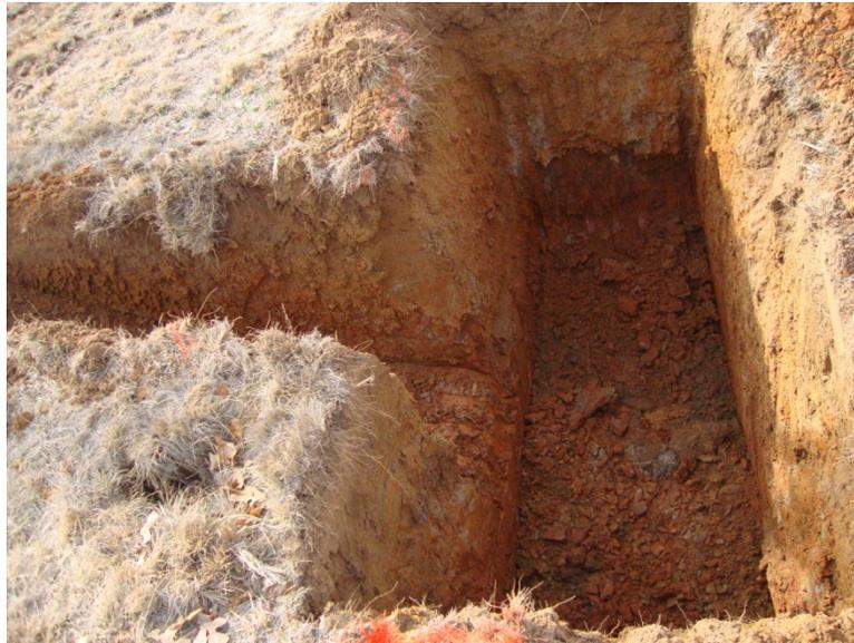
A narrow slot should be cut from the center of the long side of the hole, towards the base pad. The slot should extend from about 2' above the bottom of the hole out at a 45° angle from horizontal. This slot will be used for the anchor rod.
