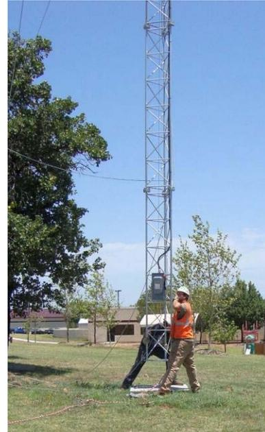
22. Set the tower down on the base pad, with the pier pin through the center hole in the bottom plate, and rotate it as necessary to properly align the guy cables with the anchors.
